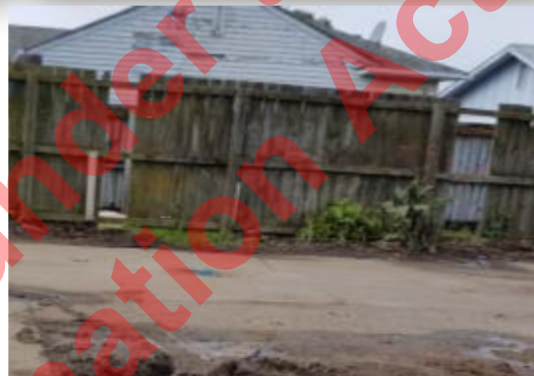
Above – Photos show existing boundary fencing with a minimum of 900mm in height and can be repaired in sections or isolated areas.
