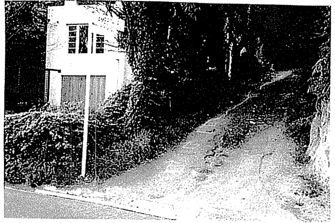
A.8 Lambeth Road - 3 properties
