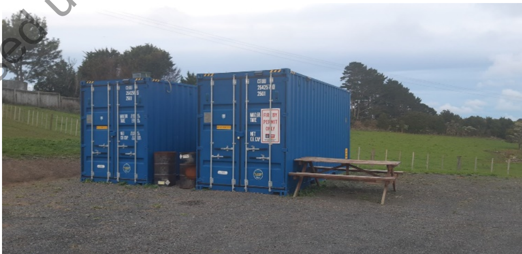
Cavalli VFB: Current fire station comprising two shipping containers on a leased site.
