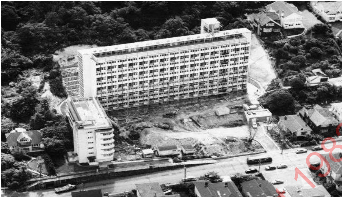
The Gordon Wilson Flats are set back from The Terrace and are surrounded by a bush back-drop below the Victoria University ridgeline. To the left front of the building are the Donald McLean Flats, a 1940s Moderne-styled block which was constructed a decade earlier.
