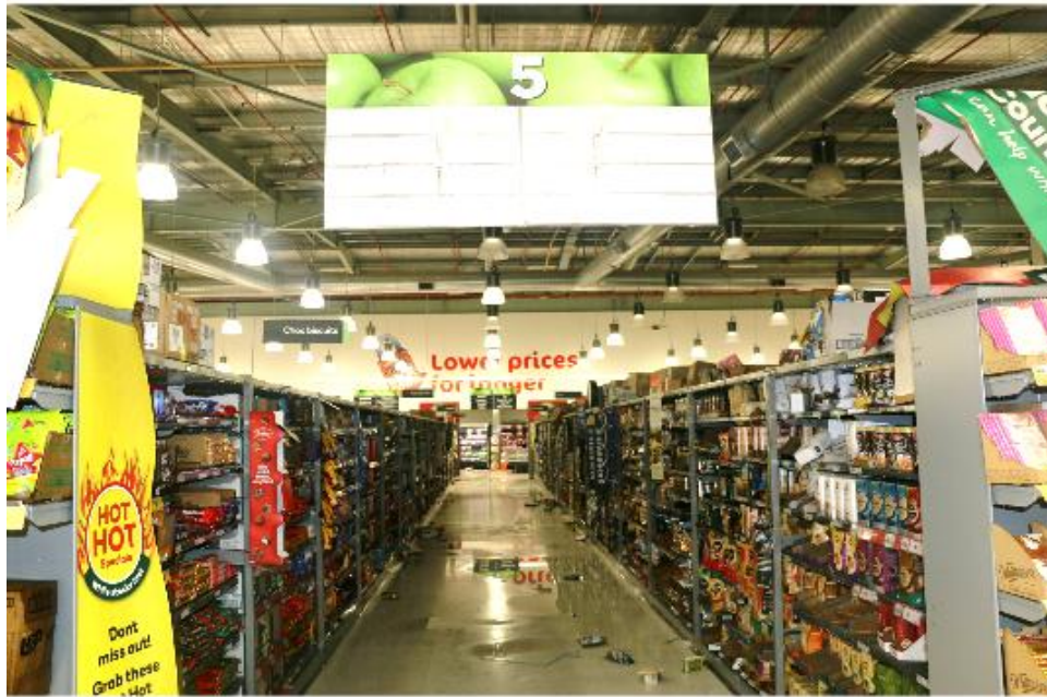
Photo 20: Aisle number 5 showing minor smoke and heat damage.
