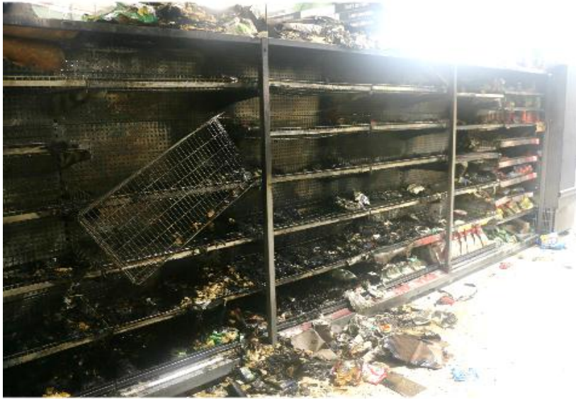
Photo 22: The section of the shelves that had the most damage in comparison to the other shelves.
