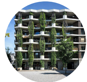
Active façade facing town square.
