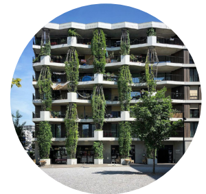
Active façade facing town square.
