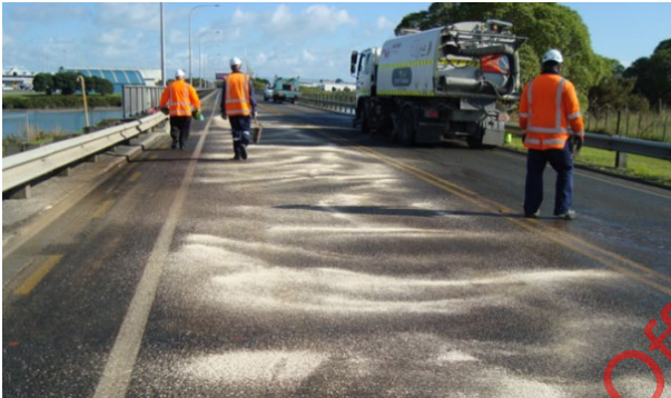
Figure 22. Vehicle fluids resulting from a crash are being removed using absorbent material and sweeper truck.
