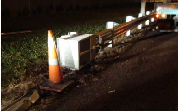
Figure 28. Energy Absorbing barrier terminal head temporarily mounted to protect damage guardrail.
