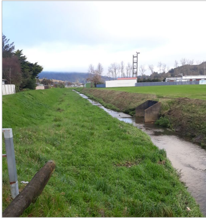
Figure 7-10 Historic Channel Improvements on left hand bank (Photo taken from Nelson Crescent Bridge looking downstream)
