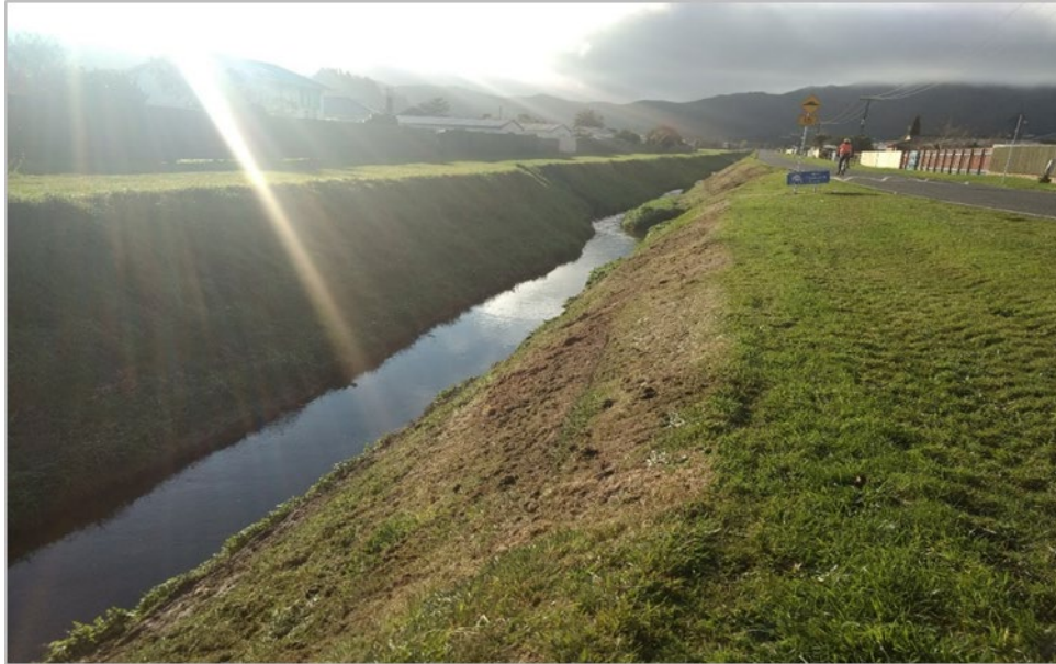
Figure 7-7 Black Creek looking upstream from Norfolk Street bridge
