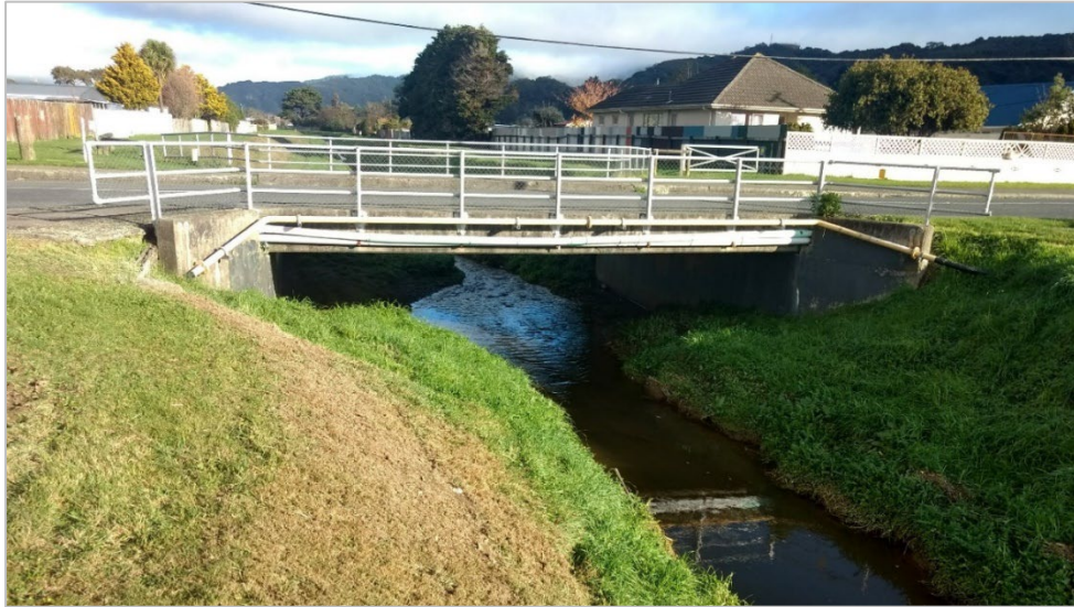
Figure 7-9 Norfolk Street bridge
