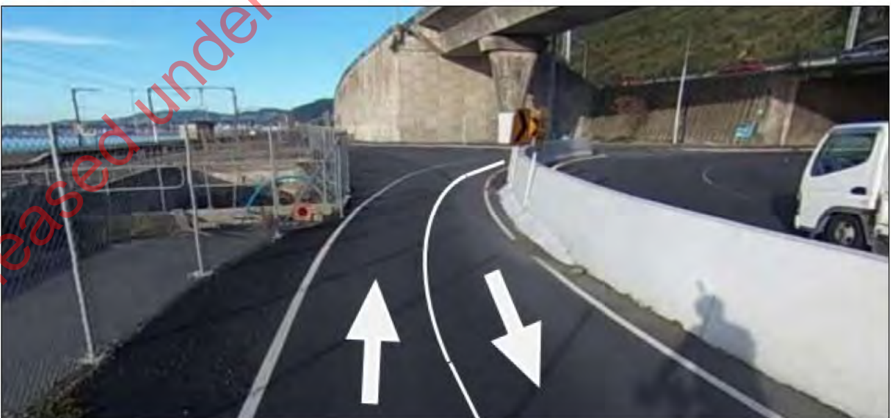
Figure 31: Shared path markings at narrow section of shared path at the motorway underpass.
