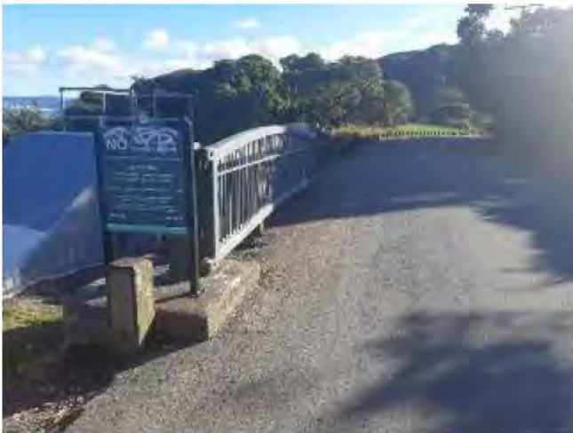
Figure 46: Hutt City Council owned and operated gate
