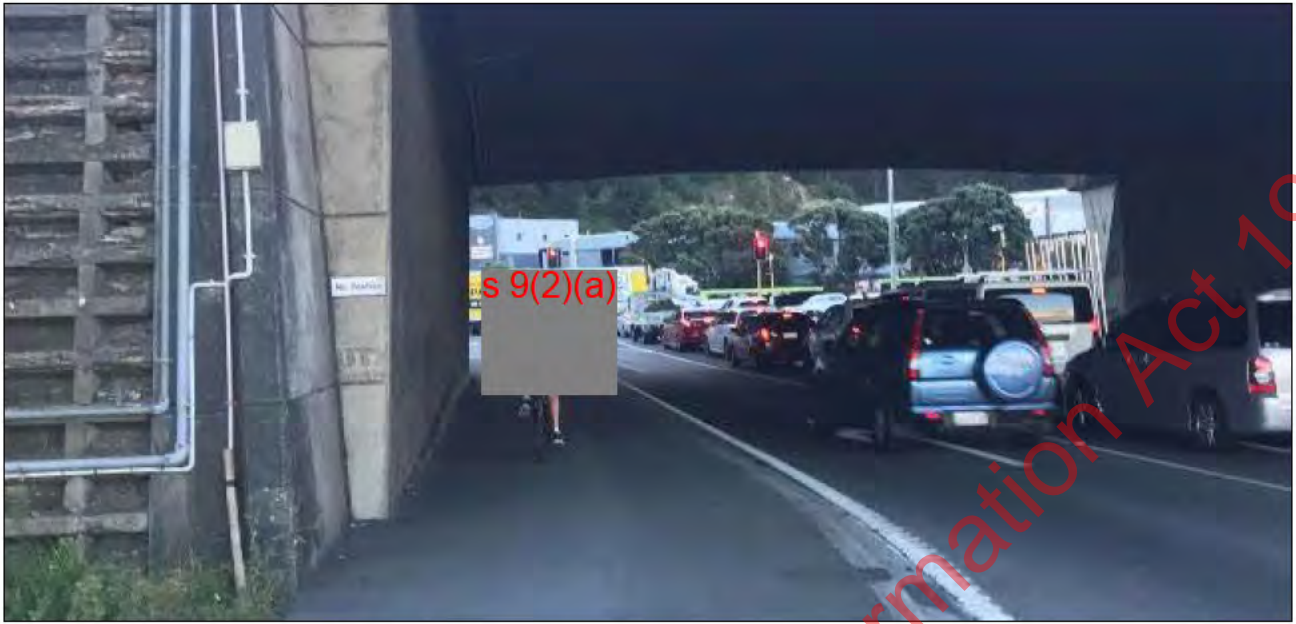
Figure 28: Narrow path through the motorway underpass tunnel.
