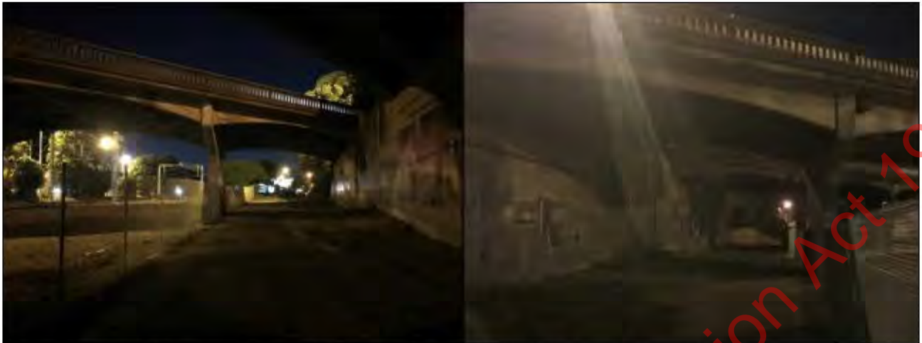
Figure 17: Limited visibility and increased personal safety risk beneath the unlit Petone underpass.
