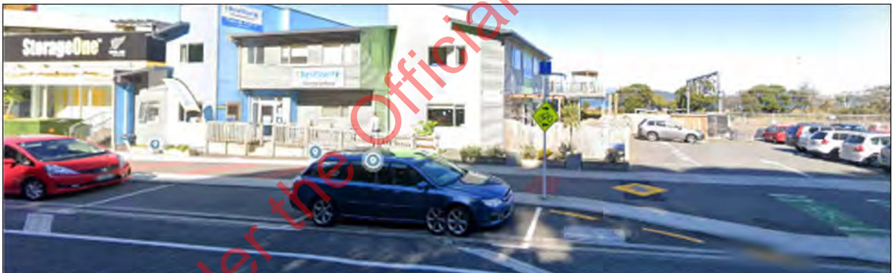
Figure 35: Existing red coloured surfacing bars at conflict zone along the Hutt Road
