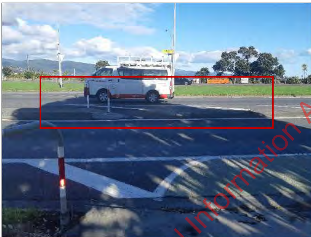
Figure 20: Current cyclist facilities for cyclists on the Petone off ramp who want to access The Esplanade or the Reserve
