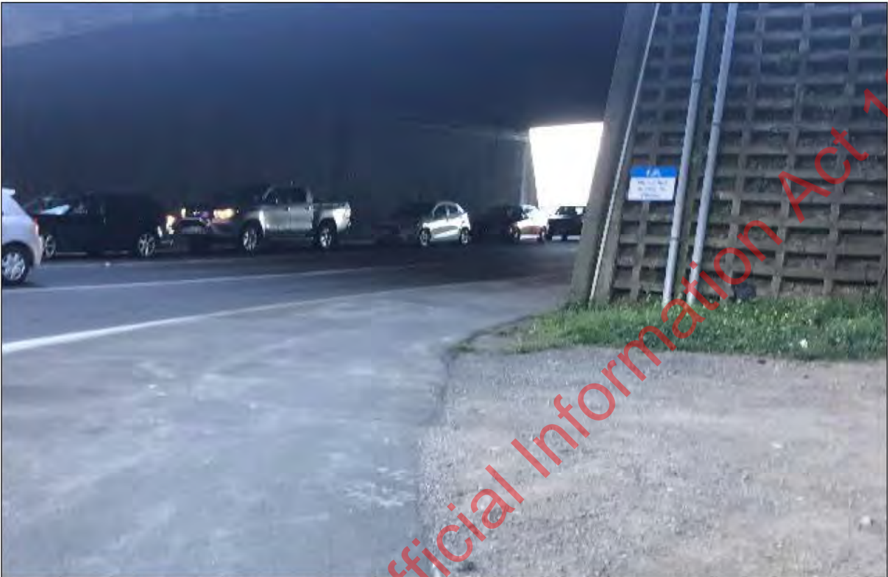
Figure 30: Limited forward visibility from the Hutt Road through the motorway underpass tunnel.
