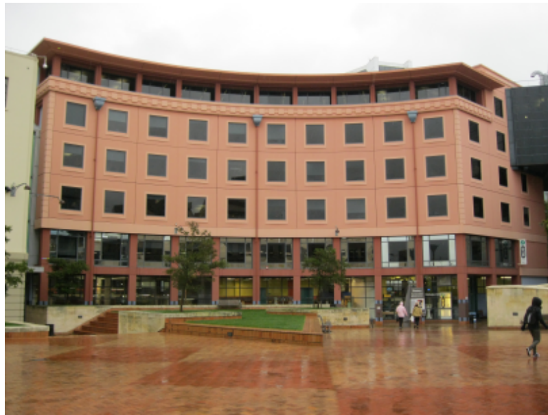
Figure 3-1: Civic Admin Building
