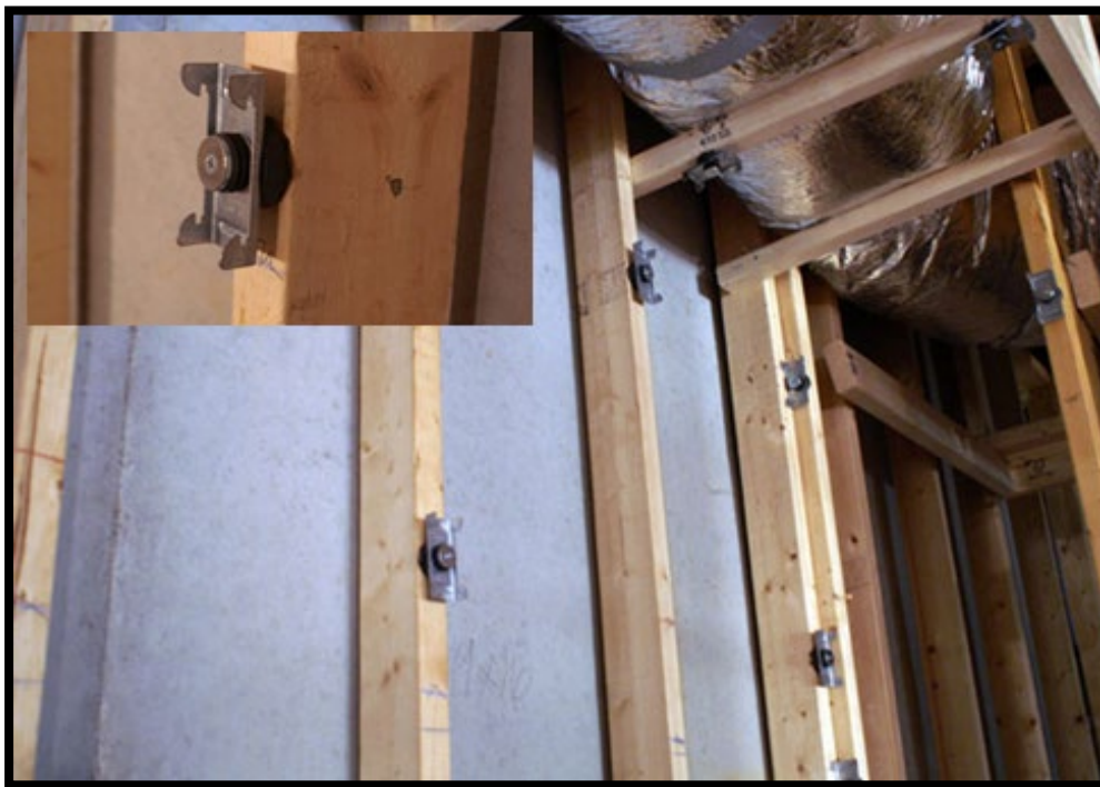
Figure above: sample of resilient clips on rubber grommets to reduce vibration. The clips are designed to carry a channel which the drywall is attached to.
