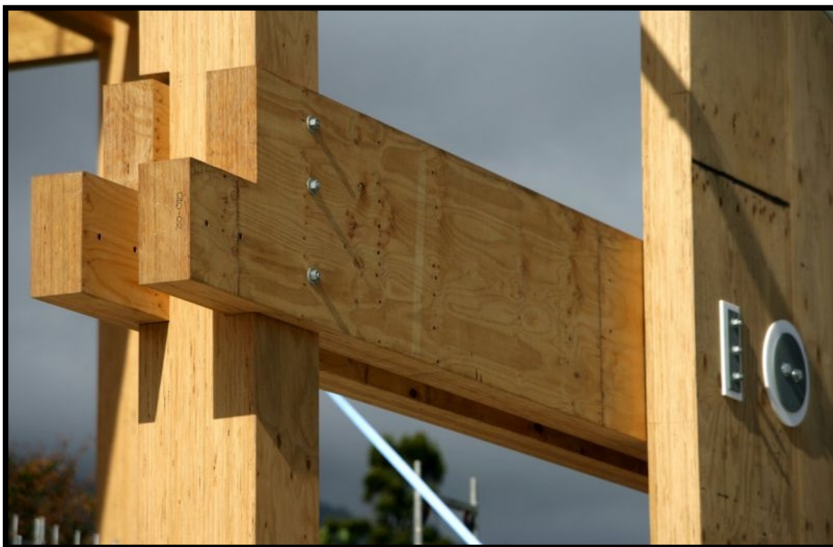
Figure 36. Sample of LVL, sourced from Nelson Pine Industries Ltd.
