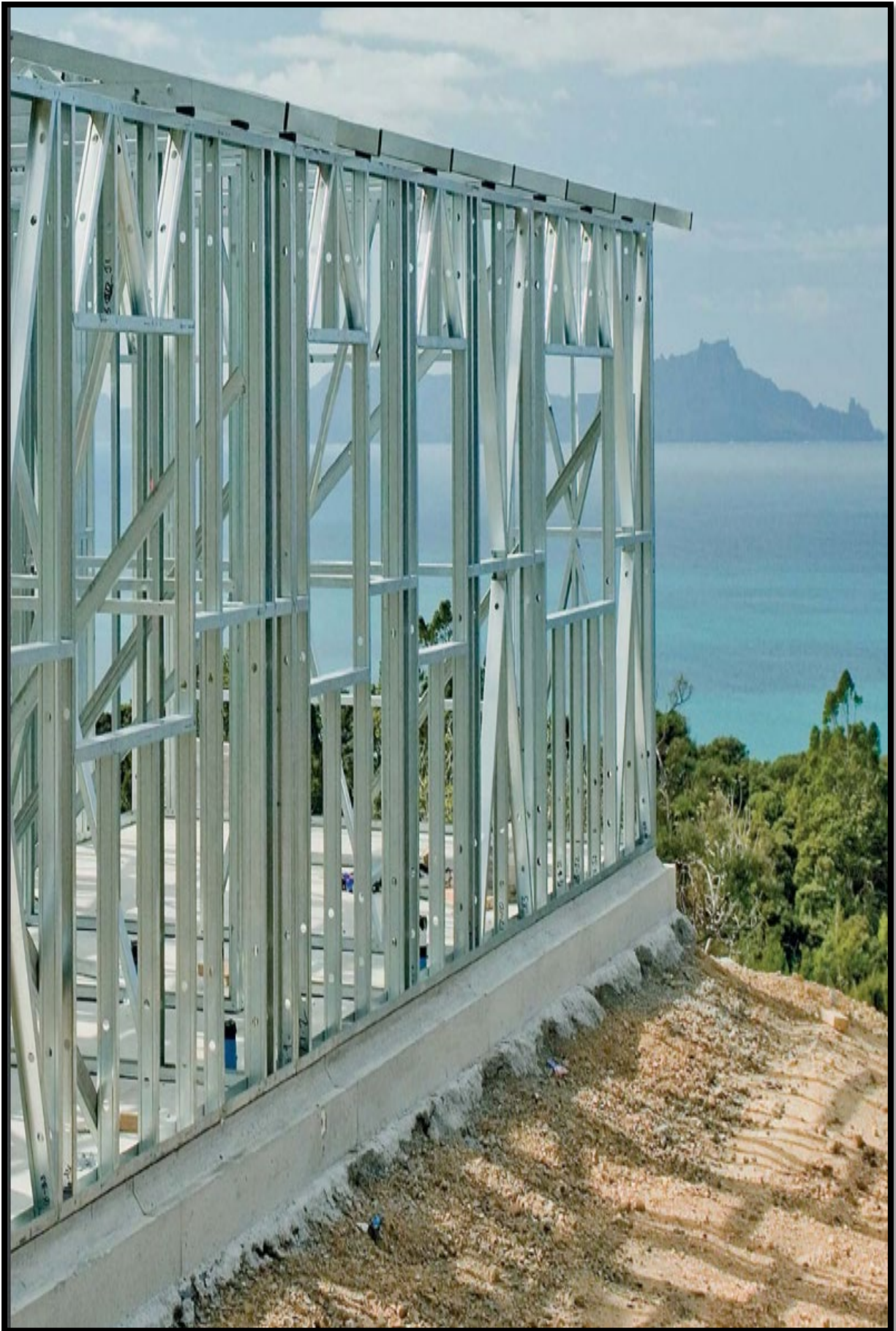
Figure 170. Sample of steel framing
