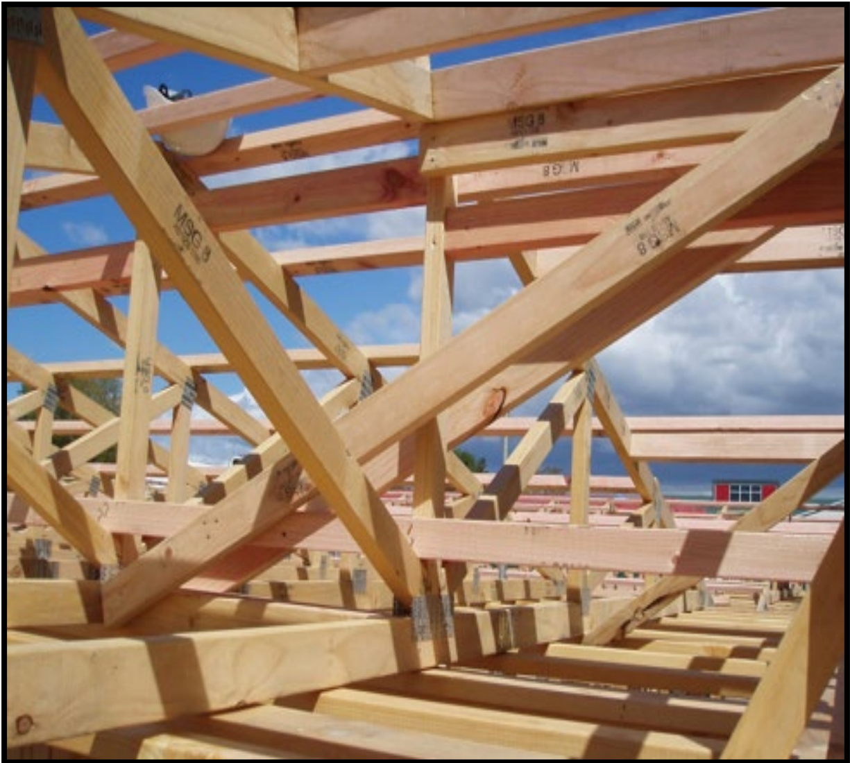
Figure 102. Sample of a roof space brace
