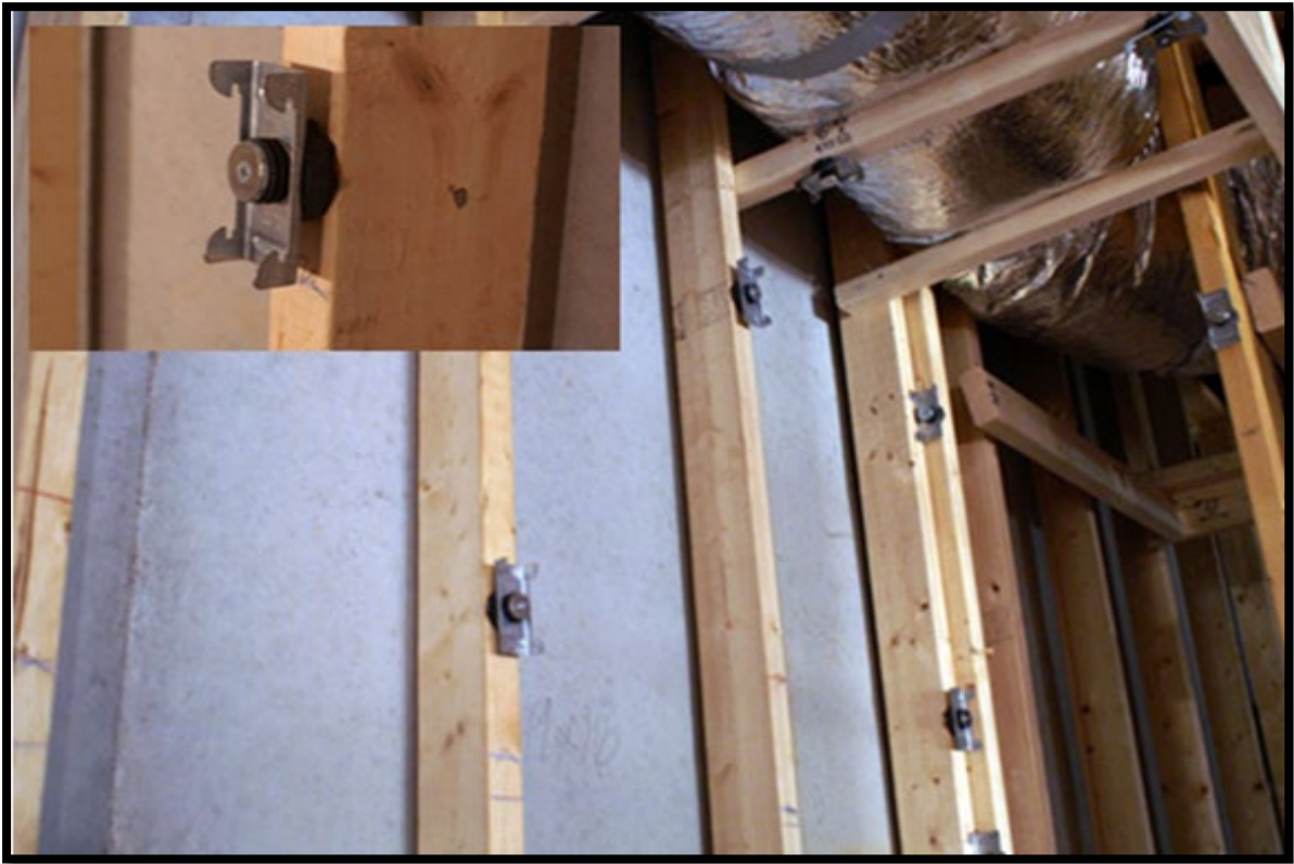
Figure 70. sample of resilient clip on rubber grommets to reduce vibration. The clips are designed to carry a channel, which the dry wall is attached to.
