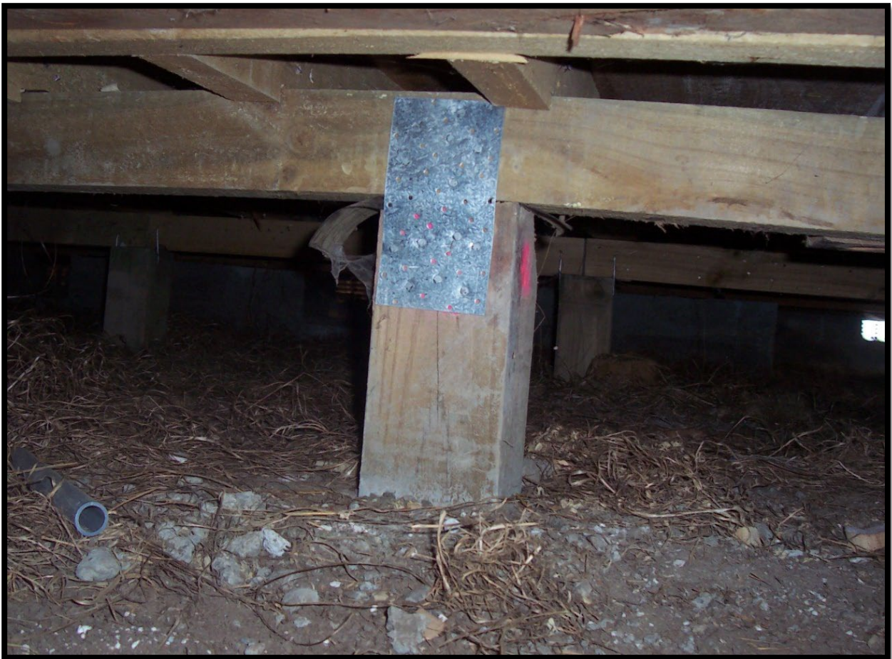
Figure 1. Sample of subfloor anchor pile and fixing.
