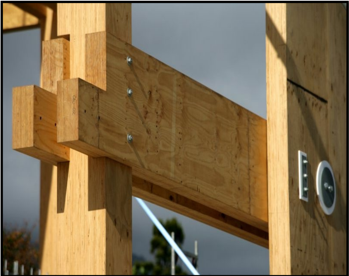
Figure 55. Sample of LVL beam.
