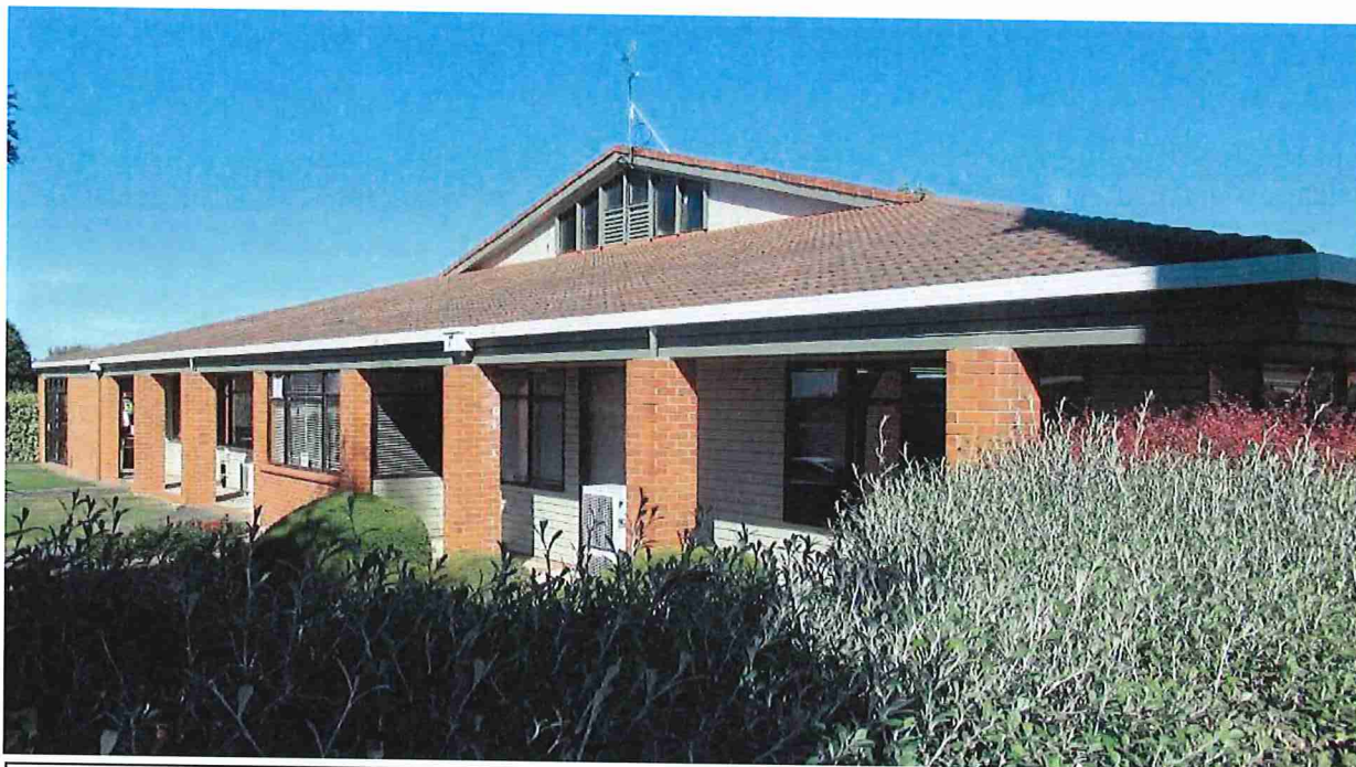
Photograph 3 – North eastern façade
