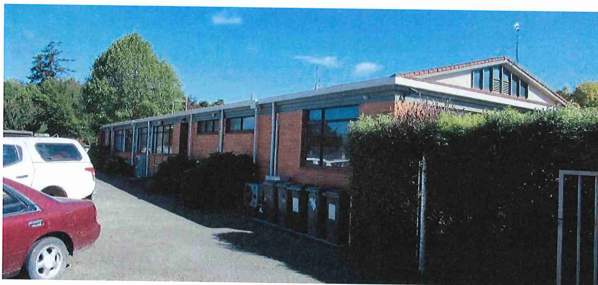
Photograph 4: South eastern façade
