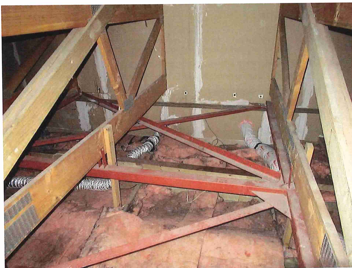
Photograph 6: Roof structure showing bracing lattice
