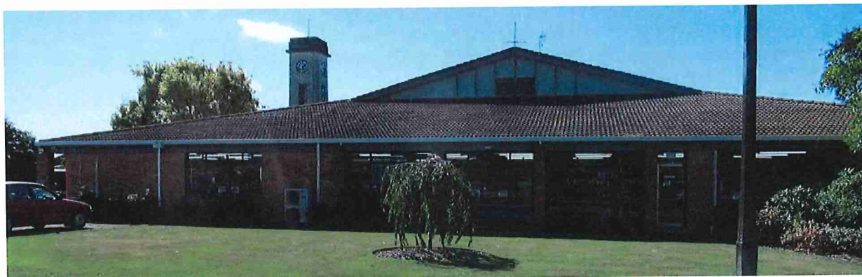
Photograph 5: South western facade
