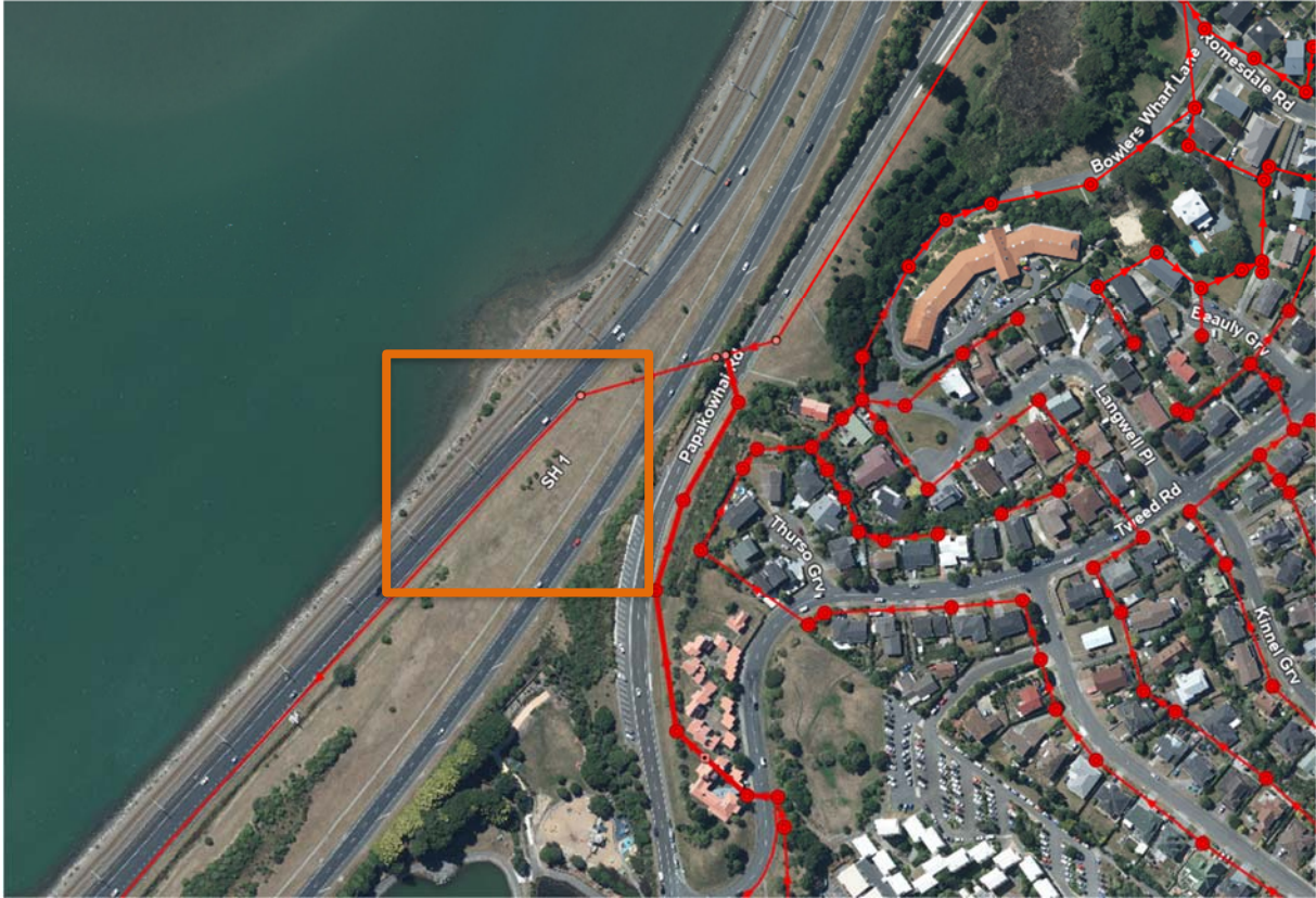
Figure 1: Pipeline Failure (shown in orange)
