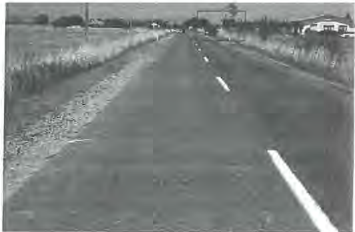
Fig 2 View east of Bush Road, 108 Bush Road is at top right corner of view with driveway in boxed area.
