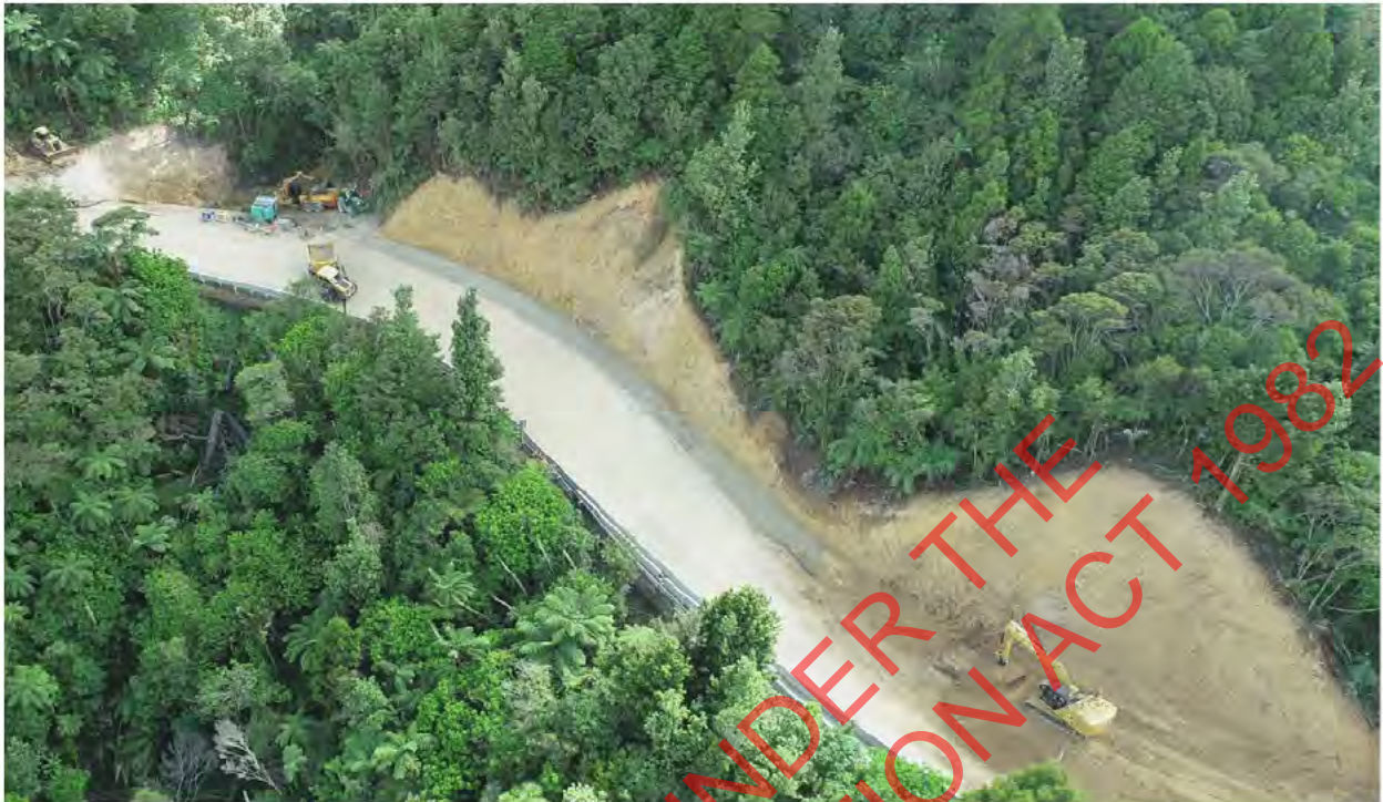
Aerial picture of work sites H, I and J
