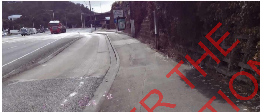
Figure 39: Indented bus facility creates a width constriction
