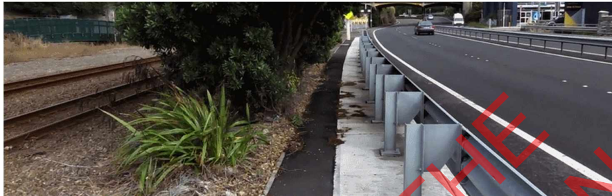
Figure 61: Limited space between guardrail and rail corridor with mature Pohutukawa trees
