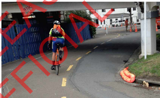
Figure 30: Centre line cuts corner
