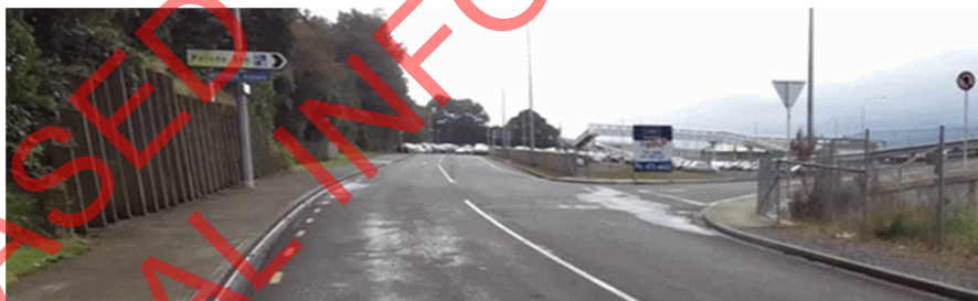
Figure 68: Retaining wall and pole constraining path width at McKenzie Avenue
