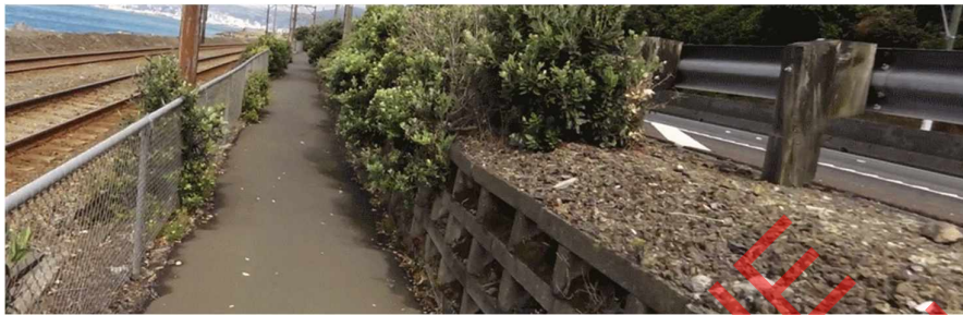
Figure 48: Road surface at head height
