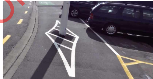
Figure 14: Pole warning markings
