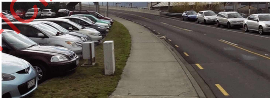
Figure 69: Service utilities adjacent to formal overflow parking area
