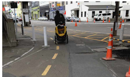
Figure 31: Centre line leads to hazard
