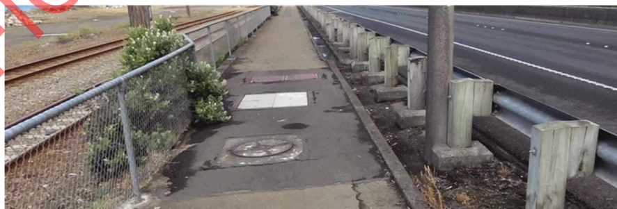
Figure 47: Fence, tree, service lids, kerb, poles and guardrail
