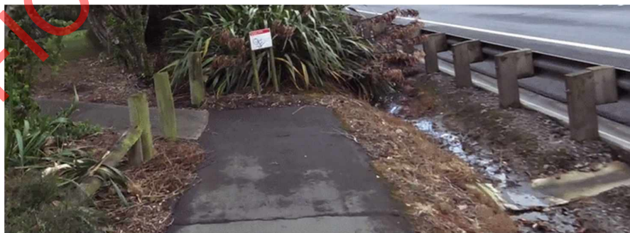
Figure 76: Tight bend with low bollards and drain
