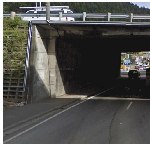
Figure 44: Underpass looking west
