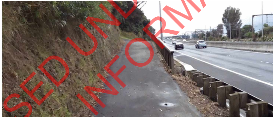
Figure 75: Steep embankment and retaining wall
