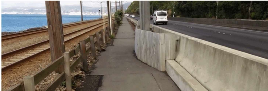
Figure 51: Narrowest section of new path at 1.18 m wide
