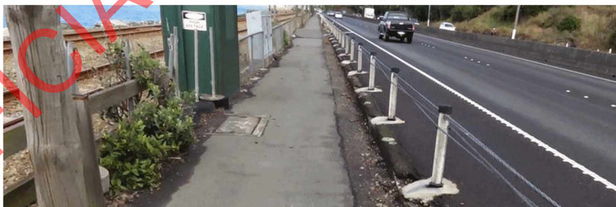
Figure 50: Fence, poles, service structures and lids, wire rope constraints
