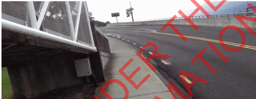
Figure 67: Restricted path width at overpass ramp
