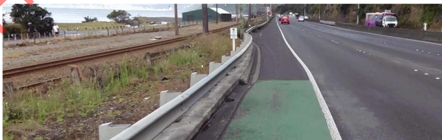
Figure 59: More space is available at CH 4,600
