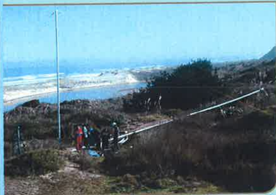
Installing the new wind mast at Waipoua.
