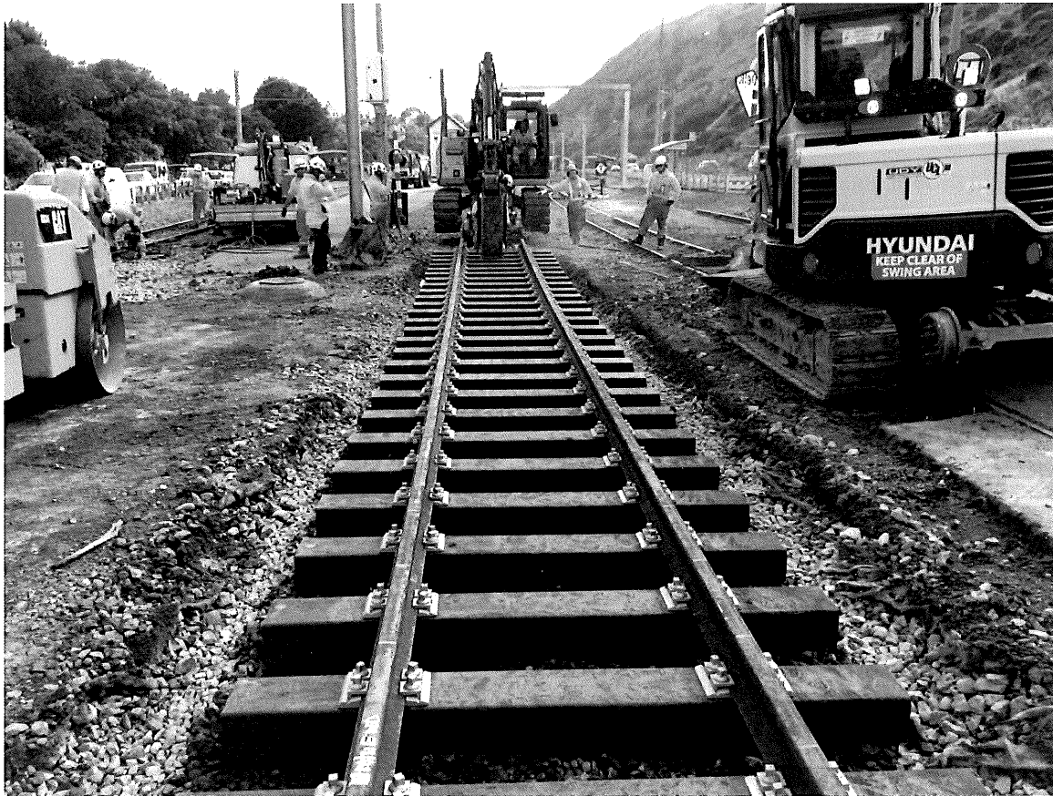
Figure 8 – New track-set being laid for Beach Road Level Crossing
