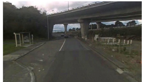
Outbound: On Hutt Road, after the intersection
