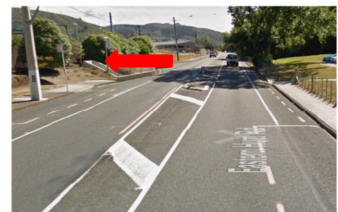
Outbound: Along Eastern Hutt Road near the station subway access
