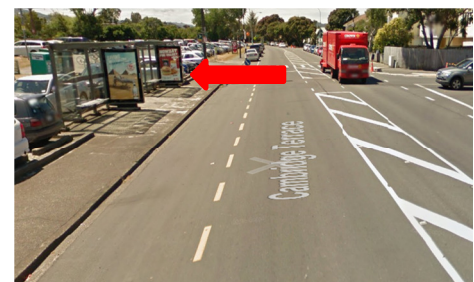
Outbound: The Cambridge Terrace bus shelter in front of the station car park
