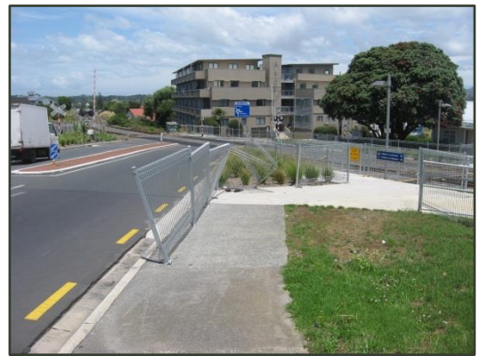
Photo 3: St Jude Street Crossing looking westward
