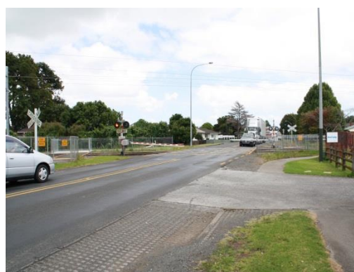
Photo 11: Manuroa Road crossing looking south west
