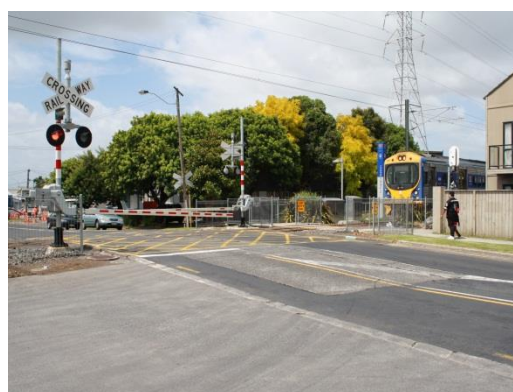
Photo 14: Mays Road Xing looking south east
