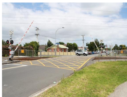
Photo 10: Taka Street crossing looking south west
