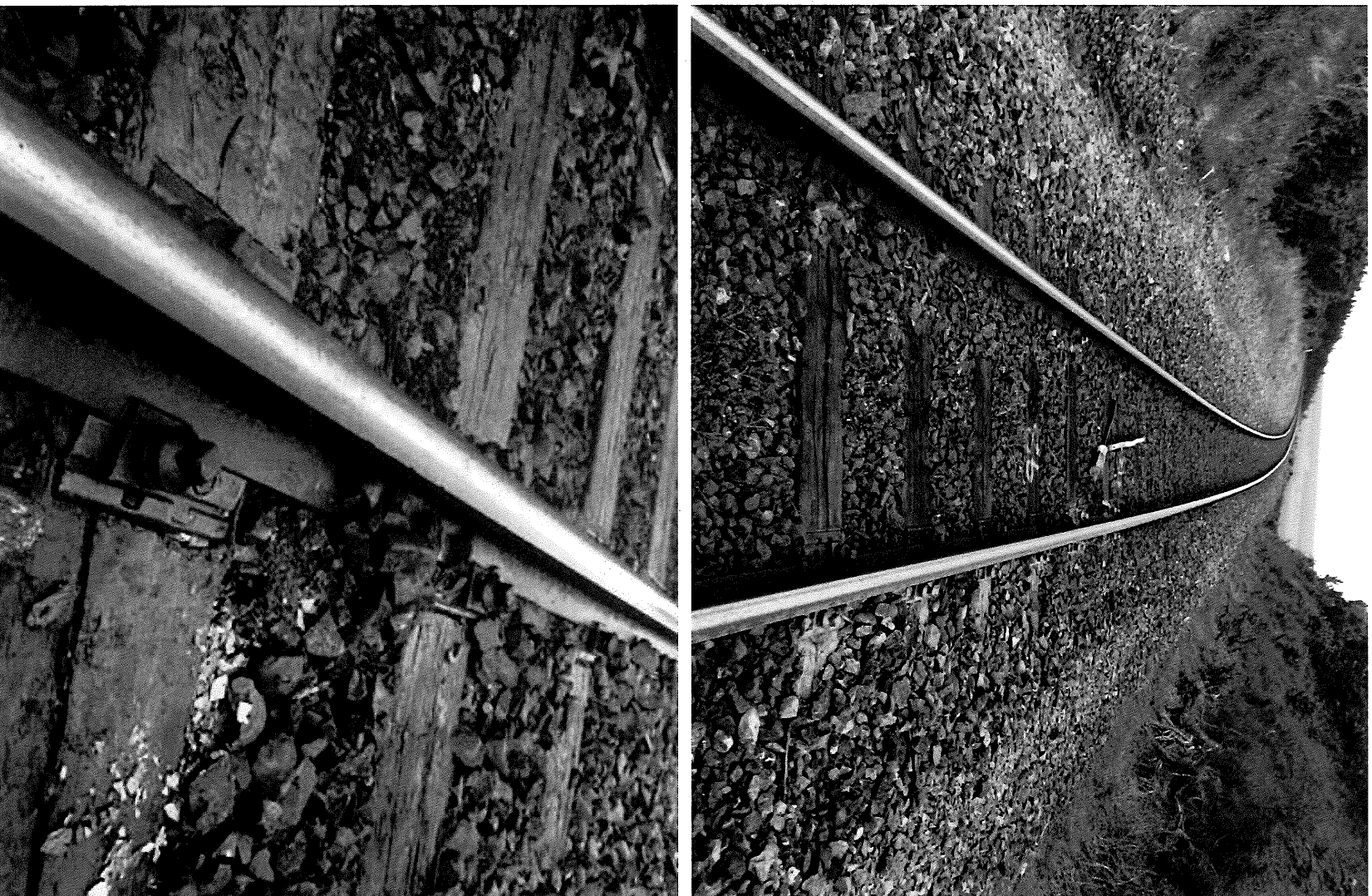
Figure 27 – End of Life and Poor Condition Track Photos
