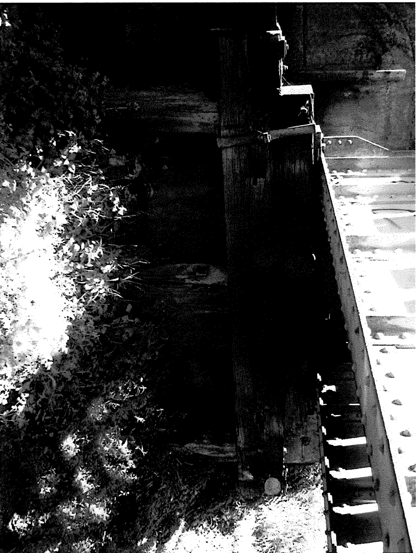
Figure 31 - End of Life and Poor Condition Piers: Br23 NIMT
