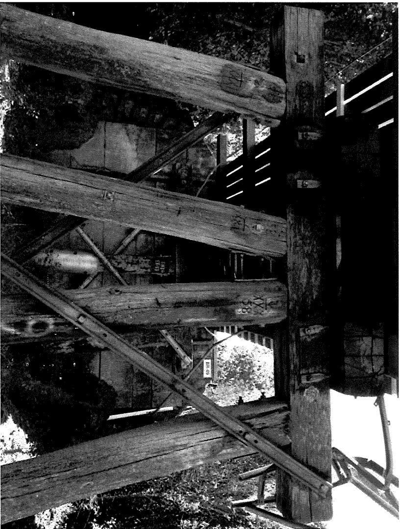
Figure 31 - End of Life and Poor Condition Piers: Br23 NIMT
