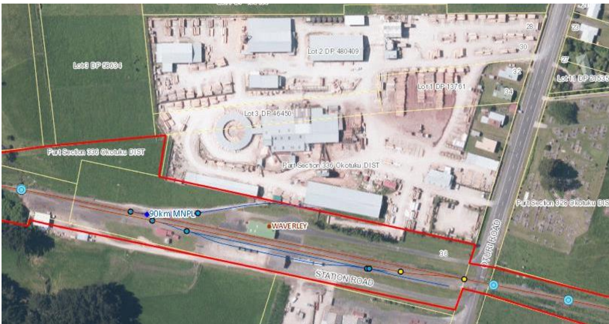
Figure 14: Aerial view of Waverley station
